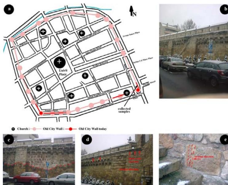
Fig. 1 – The fortress wall of Cluj Napoca, Baba Novac area, the west part of the wall: The initial wall plan (a), the west part of the wall (b), humidity due to capillarity (c), black crust (d), stratum direction perpendicular on the block orientation in the building (e).
